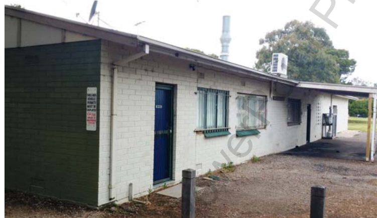
Council building GS Kingston Park / Wirraninthe (Park 23)
